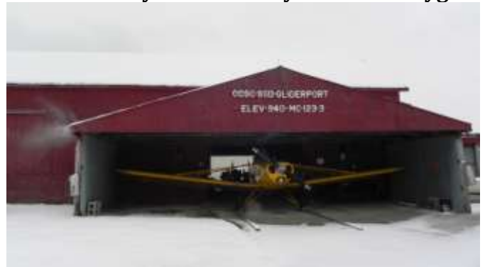
East wind clearing snow from 909's barn
